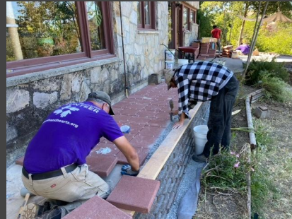
Pavers replaced old decking in Zone Zero
