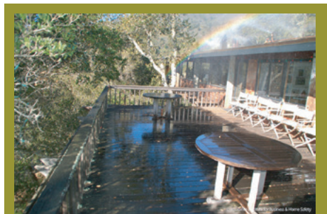
Photo 3. Roof-edge mounted sprinkler. Note these sprinklers did not deliver water in the near-home area. With this scenario, a sufficient number of wind-blown embers would have to be quenched in order to avoid ignition of the siding and decking in this zone, particularly at the deck-to-wall intersection.
