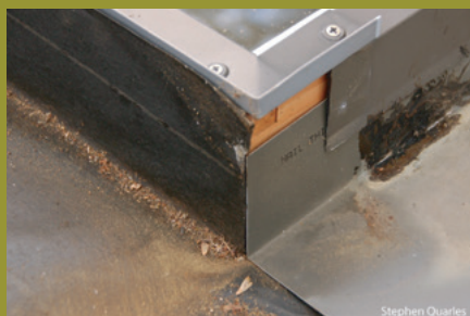
Photo 4. Metal flashing protects the framing members of a skylight from moisture, a direct ember ignition, or flames from ember-ignited vegetation debris.
