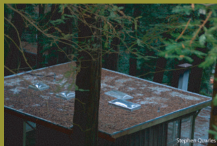
Photo 2. Minimal accumulation of vegetative debris accumulated on these dome-type skylights on this low-slope roof.
