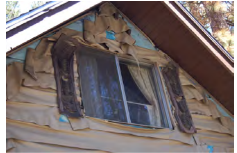
Deformed vinyl siding from a radiant heat exposure from a nearby burning home. Source: Stephen L. Quarles
