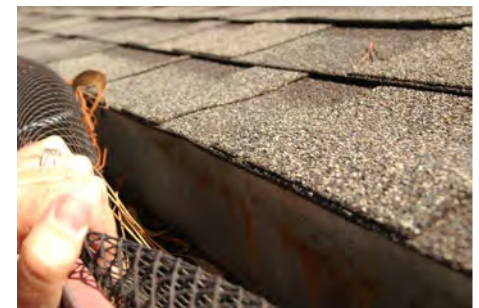
Gutter with integrated drip edge. Source: firecenter.berkeley.edu/bwmg/gutters.html
