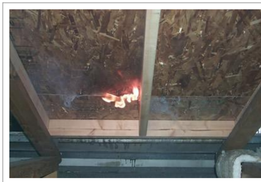
Flame-through to the underside of a roof deck. This roof covering failed, so as constructed, this is not a Class A roof.
